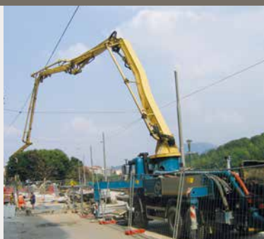
Pompaggio CLS alleggerito a base di Pomical / Pumping of lightened concrete having as basis Pomical
