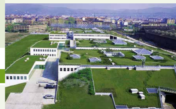
Sistema Vulcaflor per tetti verdi Vulcaflor system for green roofs ENVIPark, TORINO
